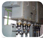
Power sensitive equipment
